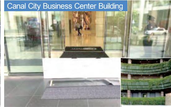
In contrast to the existing water stops of +50 cm from the standard level, (\*) the new water stops are +100 cm from the standard level, enhancing the anti-inundation function,
