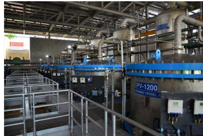
Ceramic membrane filtration facility (CeraMac®) that started operation
