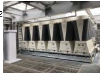
Installation of high-efficiency heat-source system (Shin-Yokoyama TECH Building)
