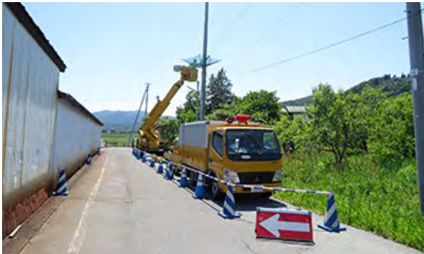
Placing safety barriers around the work area
