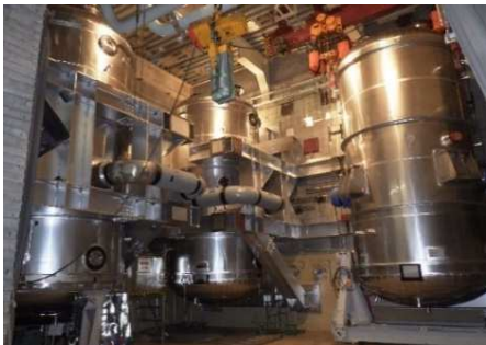
Onagawa Nuclear Power Station undergoing construction work for safety measures (Venting equipment for containment vessels with filters)
