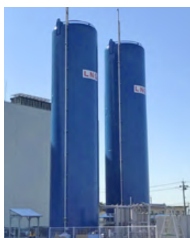
LNG storage tanks (Two tanks with capacity of 100 kL each)
