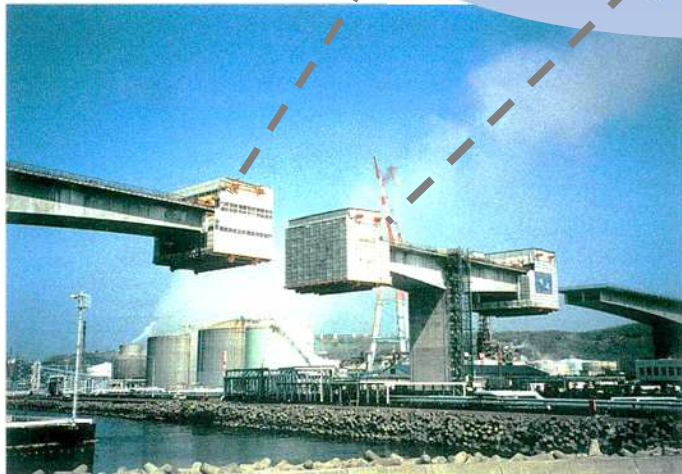
Illustration of overhanging erection method for girder bridges
