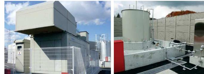
In preparation for natural disasters and other emergencies, our 21 distribution centers across the country are equipped with emergency power generation facilities that are capable of supplying power for up to 72 hours.
