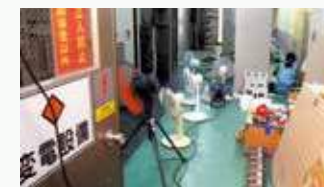
Restoration work while drying a submerged electric room with fans
