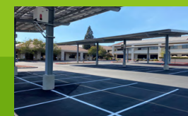
Solar panels installed in carports
