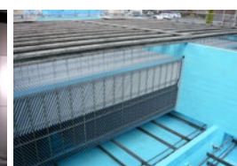
Filtration and Inclined Plate Settler
