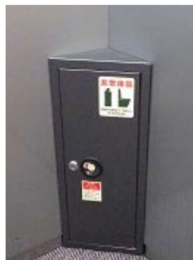
Elevator emergency goods box (Daiwa Azabu Terrace)
