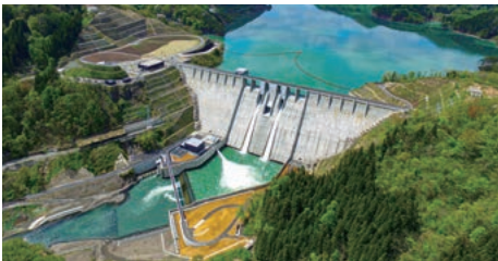
Tsugaru Dam (Aomori Prefecture) 2016 Positioned as the redevelopment of the Meya Dam located 60 meters upstream, this multipurpose dam used a cruising roller compacted dam-concrete method to shorten the construction period. Japan Society of Civil Engineers Civil Engineering Design Grand Prize 2018, Japan Society of Civil Engineers Outstanding Civil Engineering Achievement Award 2017
