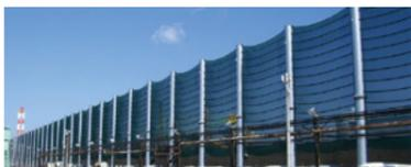
A windbreak net is installed to reduce the strength of wind and restrain the scattering of raw materials.
