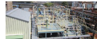
Fine undissolved matter is coagulated into bigger masses by chemical treatment, permitted to settle, and is removed.
