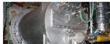
Burners featuring reduced levels of NOx generation and outstanding fuel savings have been installed.
