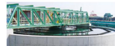
Undissolved residue from rainwater is coagulated and eliminated.
