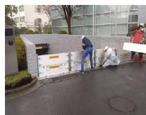
(a) Removable watertight panels
