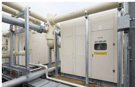
Two highly efficient, natural chiller units
