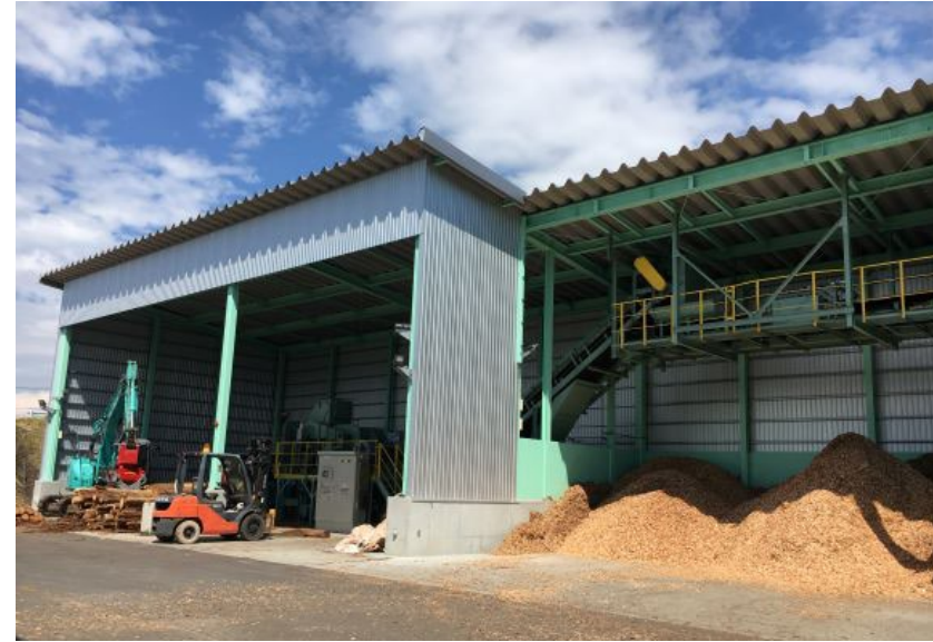
Woodchip factory incorporated into Nishiki- machi 2 MW Woody Biomass Power Plant
