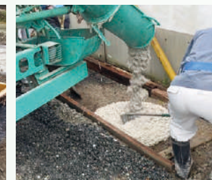
Placing (agitator car's shoot)
