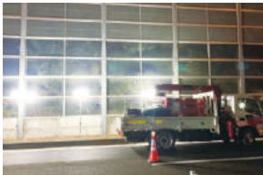
Comparative Investigation of GTL Versus Diesel in Terms of Fuel Efficiency when Used in Lighting Generators (Chubu Branch, Kachigawa Yamada Worksite Office)
