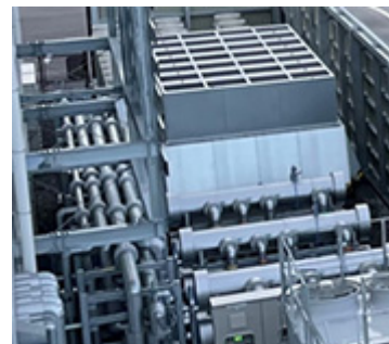
Chiller that improves energy efficiency by dividing the system into two temperature zones for different applications
