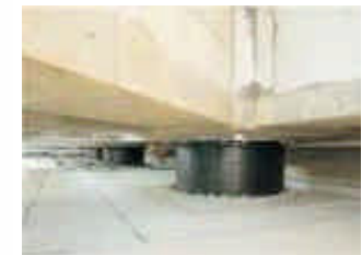
Seismic isolators
