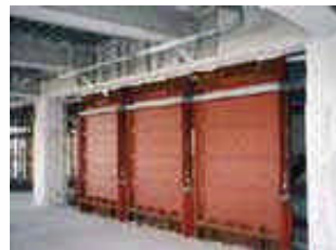
Viscous seismic damping wall
