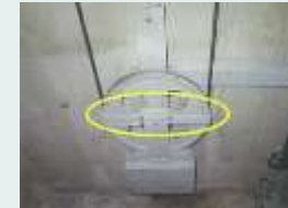
Rope misalignment stop
