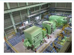
Exhaust heat recovery system at Kanda Factory
