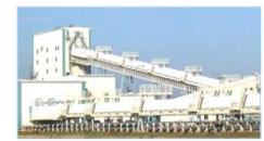
Storage and conveyance machinery for coal-fired power plants (air floating conveyors, unloaders, siloes)
