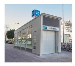
Tokyo Metro Co., Ltd. is installing a total of 10 Waterguard Waterproof Shutters at three subway stations in Tokyo (Kanamecho, Asakusa, Suehirocho). Installation of the shutters began in February 2017. During flooding, the waterproof shutters can quickly be lowered with the press of one button to prevent the inflow of surface water, and can withstand flood heights of up to 2.5 meters.
