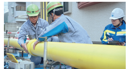
Preparing to bury an earthquake-resistant gas pipeline made of polyethylene
