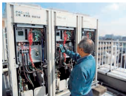
Regular inspection of air-conditioning equipment for preventing fluorocarbon leakage
