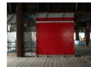
Viscous seismic damping wall
