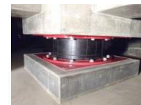
Seismic isolators
