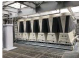
Installation of high-efficiency heat-source system (Shin-Yokohama TECH Building)
