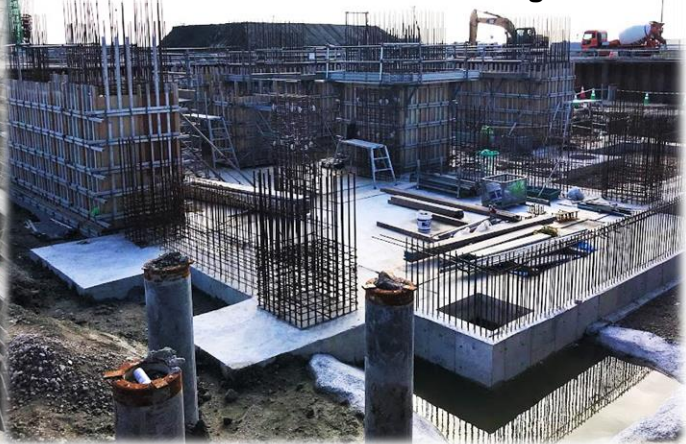
Foundation work of turbine building
