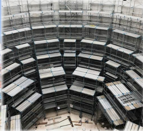
Fuel tank internal scaffolding
