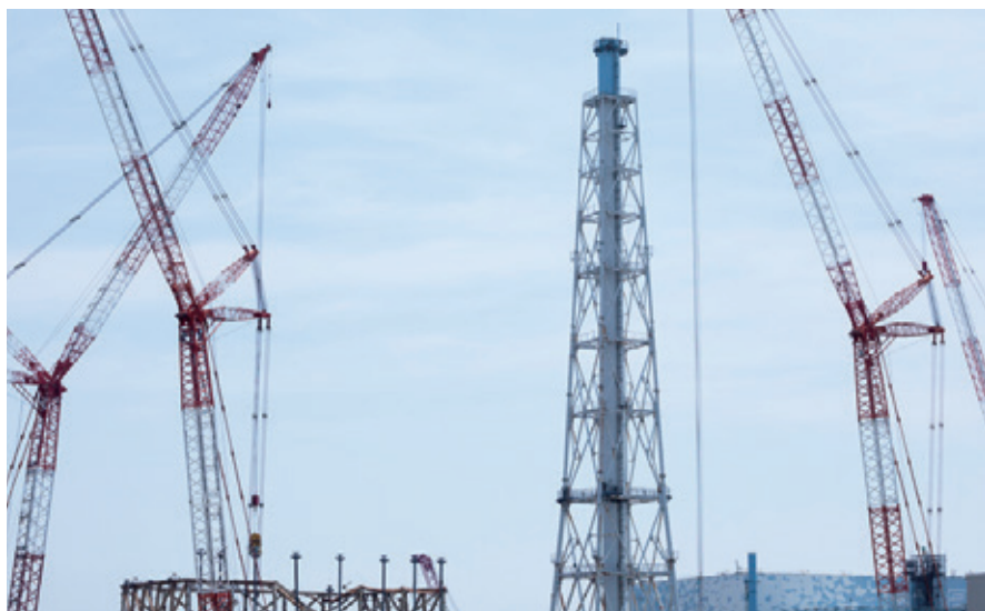
Commencement of dismantling of approximately half of the Unit 1/2 exhaust stack so as to widen seismic-resistance margins (August 2019)
