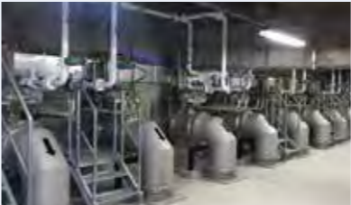
Valve room for high-speed filtration equipment
