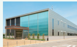
Lume Carbo system panel materials providing natural lighting, heat insulation, lightness and high rigidity
