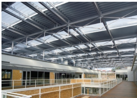
Picture of Polycarbonate Folded Plate Installation (Ceiling section)
