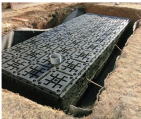
"Rain Save N" Rainwater Storage and Infiltration Tank
