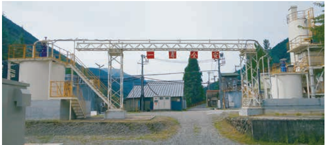
The newly installed milk of lime supply equipment and emergency generators
