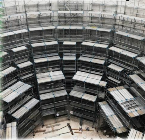
Fuel tank internal scaffolding
