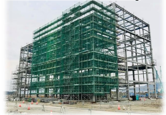
Steel construction of turbine building
