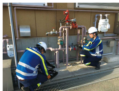
Inspecting the gas supply equipment (emergency shut-off valves)
